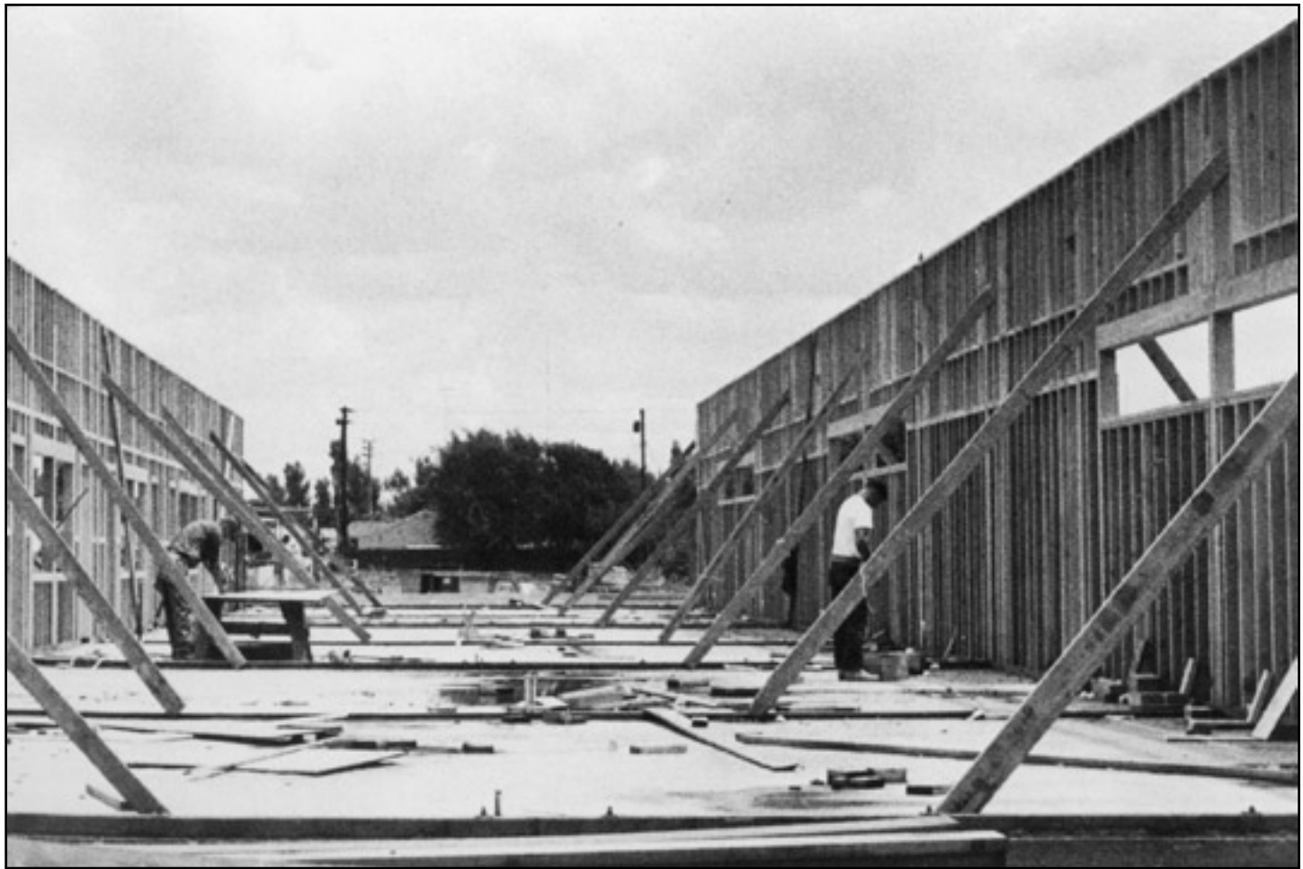
The current site of St. Francis High School is shown under construction in this c. 1963 photograph.
