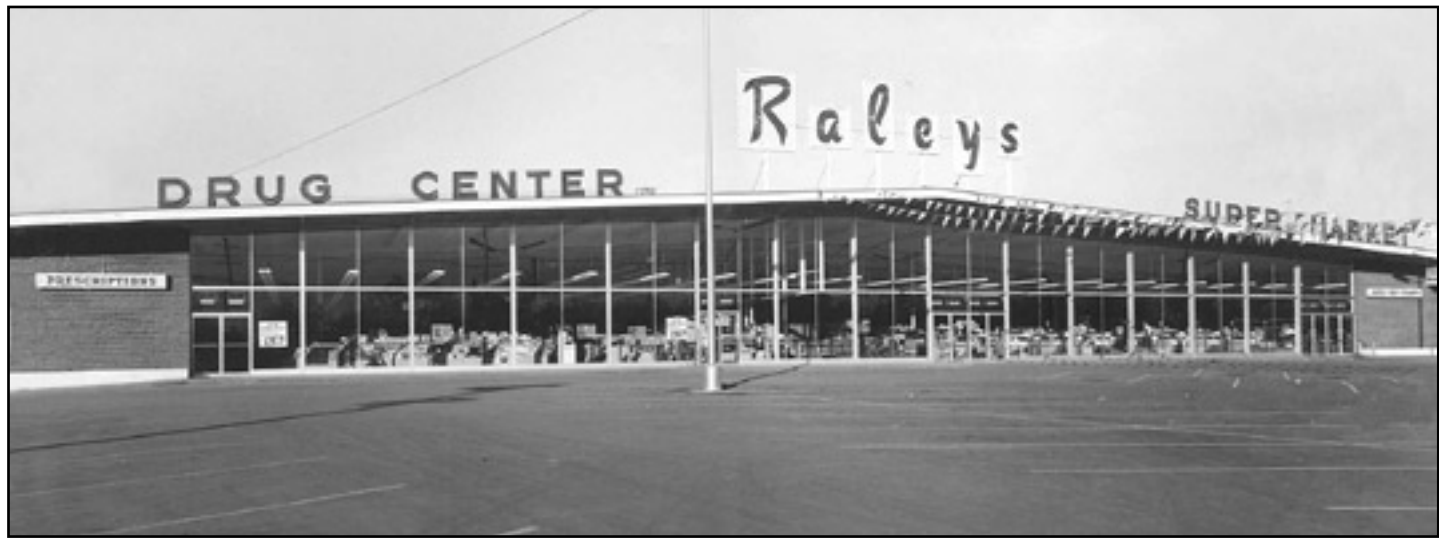
Raley's supermarket at 4850 Freeport Blvd. is shown in this c. 1958 photograph.
