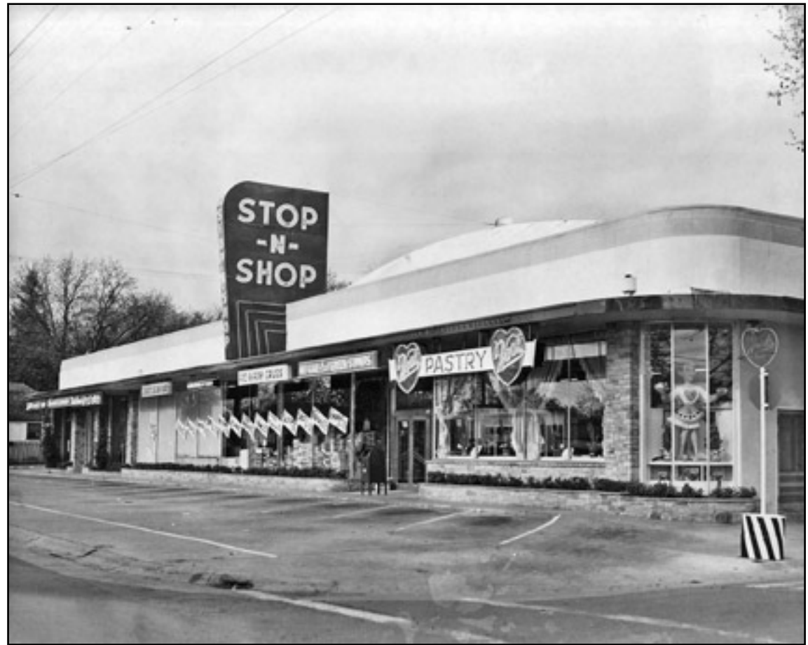
Photo courtesy of the Kassis family The Stop-N-Shop market at 3231 Riverside Blvd. served the community from 1947 to 1975. The building, which still exists today, was later home to Walter Kassis' Big K Market, which closed in 1982.
