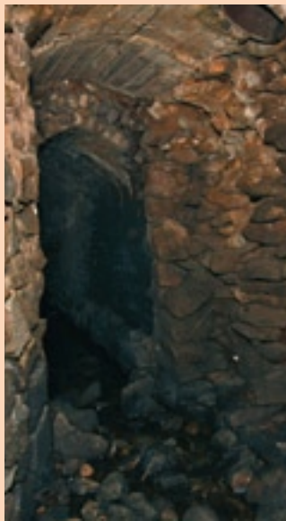
Tunneling under Folsom See page 17
