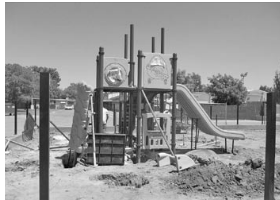
A new playground is under construction at La Sierra Community Center and expected to open to the public on Aug. 15. Courtesy photo
