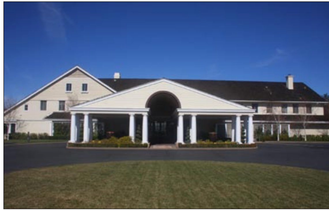
Del Paso Country Club at 3333 Marconi Ave. was established in 1916. Shown in this photograph is the site's historic clubhouse. Photo by Lance Armstrong
