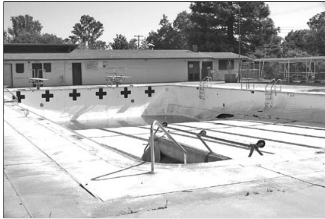
The Carmichael Park pool is shown in its abandoned state in this 2009 photograph.
