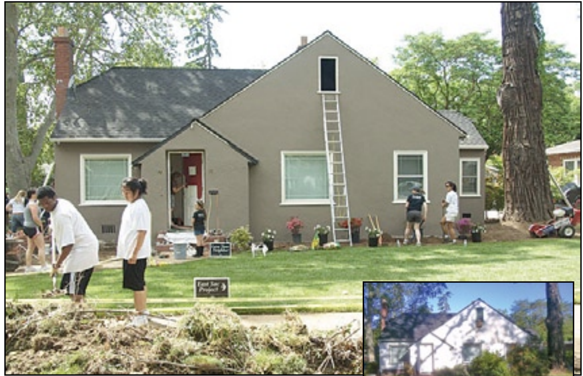
Photo courtesy Over the course of four days last month, Restoration Life Church of Sacramento remodeled the East Sacramento home of Dale and Nichelle Snapp. Pictured here are shots of the home before, inset, and after the work.
