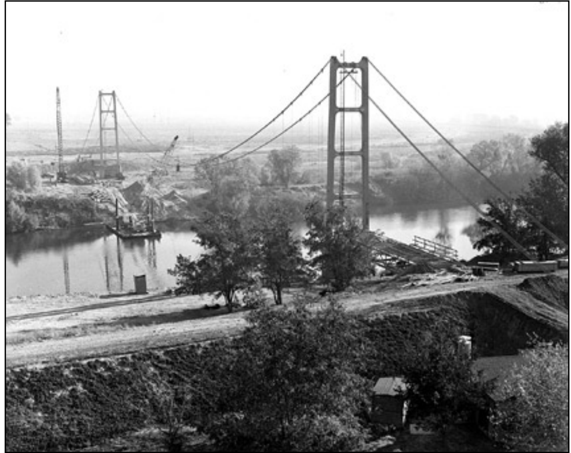
The Guy A. West Memorial Bridge is shown under construction in this 1966 photograph.
