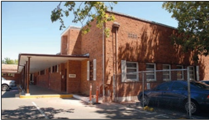
The old Sacred Heart Parish School in East Sacramento is being demolished to make way for a parking lot to support a new wing at Mercy General Hospital.
