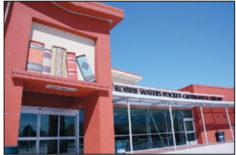
East Sacramento News photo by Danny Kam The LEED-nominated library opened Aug. 28 and cost $15 million to build.
