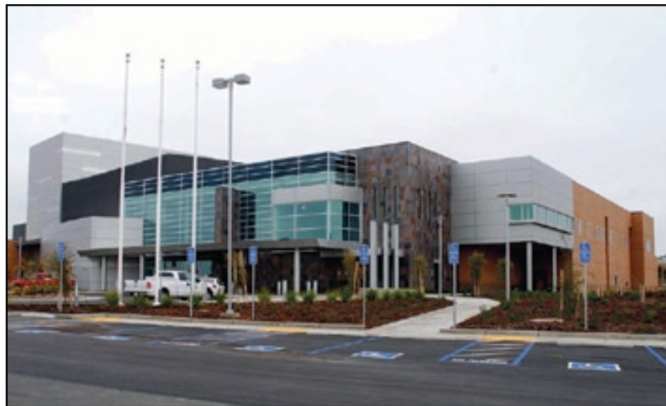
East Sacramento News photo, Tom Paniagua The Los Rios Community College District's latest facility, Three Stages at Folsom Lake College, benefited from construction during a down economy. The district was able to build more within the project's budget than might otherwise have been the case.
