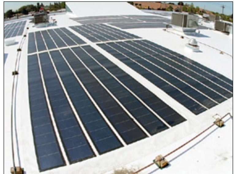
PHOTOVOLTAIC PANELS will be placed on the rooftops at St. Francis High School this winter. In this photo, flat solar panels integrated with "cool roof" technology at another location in the Sacramento area achieve increased energy savings in a commercial building.
