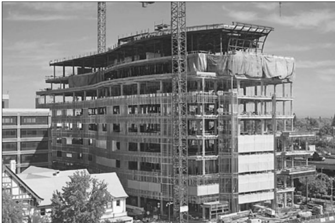
VIEW OF THINGS TO COME. The Anderson Lucchetti Women's and Children's Center, shown under construction, will replace East Sacramento's Sutter Memorial Hospital. The top level of the 10-story structure will feature a life-saving helistop for severely injured and sick patients.
