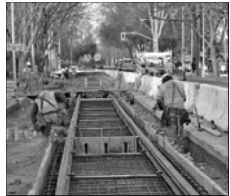
Photo courtesy, Sacramento Regional Transit BE CAREFUL. The wires are now "hot" above the new tracks on 8th Street in Sacramento. Construction continues on the RT Green Line Extension, slated to open in 2012.
