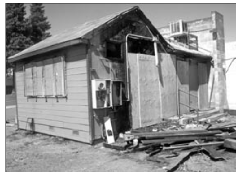
Photo by Lance Armstrong A fire occurred at the old Squeeze Inn on Fruitridge Road on May 14. Shown in this recent photograph is the back of the building, which reveals the majority of the structure's exterior damage caused by the fire.
