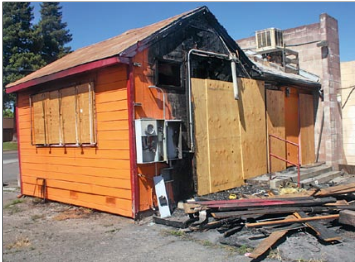
A fire occurred at the old Squeeze Inn on Fruitridge Road on May 14. Shown in this photograph is the back of the building, which reveals the majority of the structure's exterior damage caused by the fire. Squeeze Inn was founded in East Sacramento. Photo by Lance Armstrong
