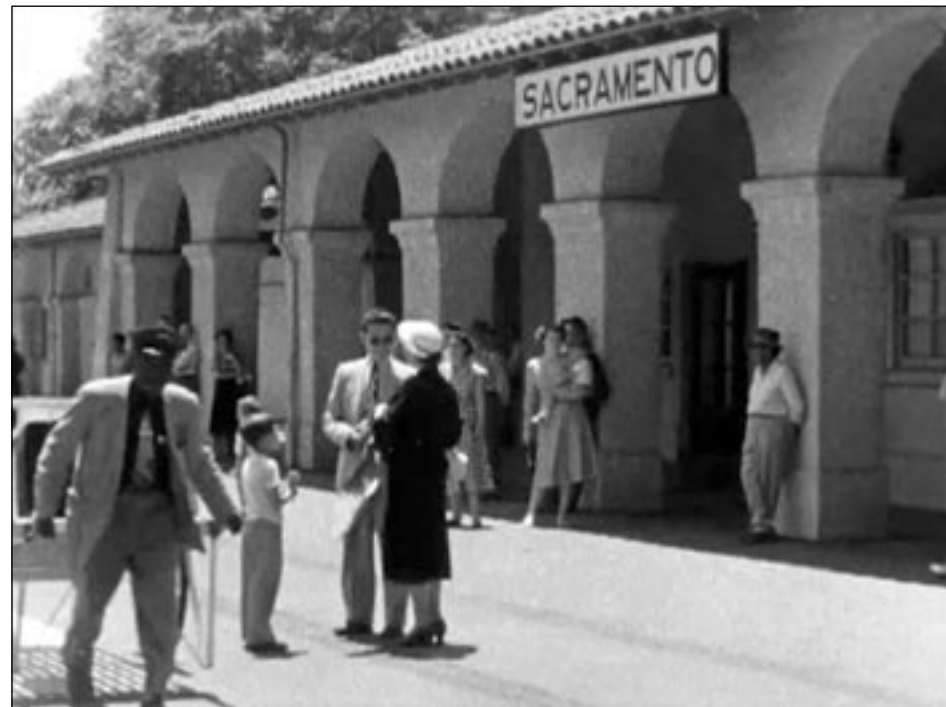
Photo courtesy of Center for Sacramento History A still image taken from an old Sacramento film shows the Western Pacific depot, which is presently home to The Old Spaghetti Factory restaurant at 1910 J St.
