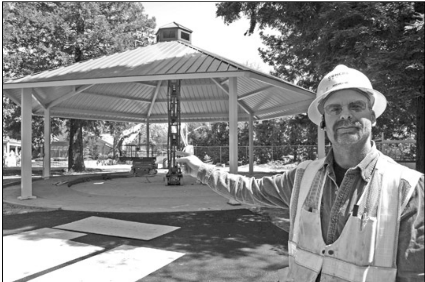
Jeremy Melton of Concrete Services points to the "in progress" construction of the Conservation Carousel at the Sacramento Zoo.
