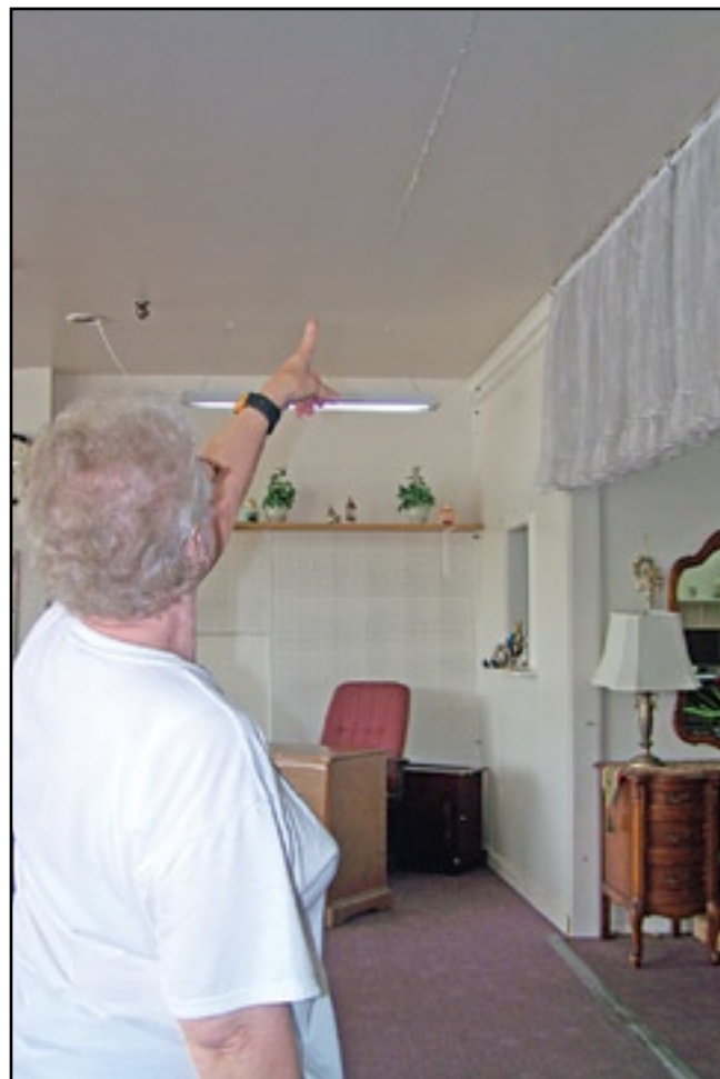
Land Park News Photo/Ryan Rose Comfort Zone office manager Helen Burgess points to water dripping from the ceiling of her office at 4420 Del Rio Rd.
