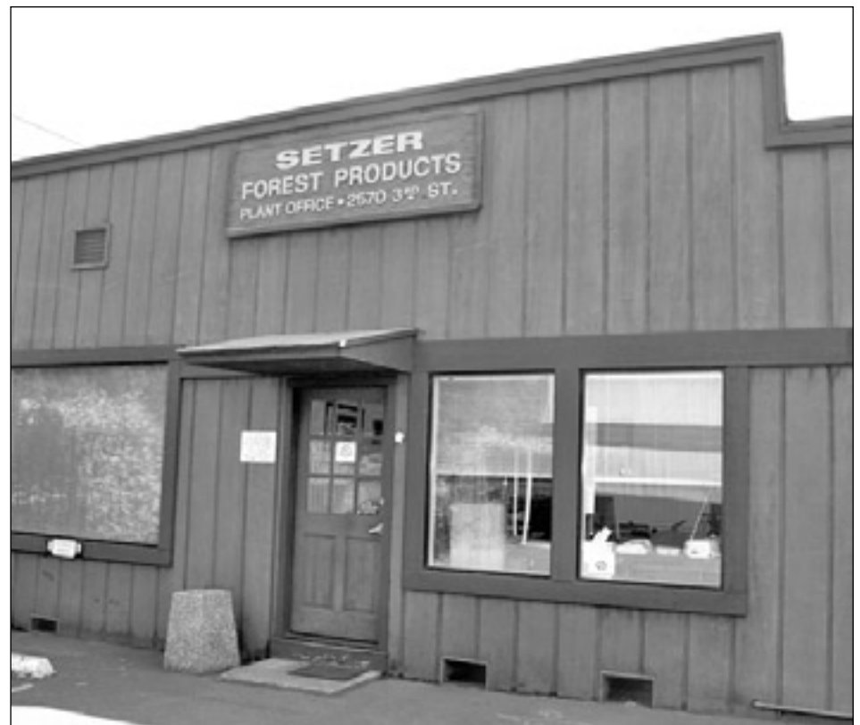
The Setzer Forest Products plant office at 2570 3rd St. is shown in this recent photograph. A portion of this structure was built in 1927.
