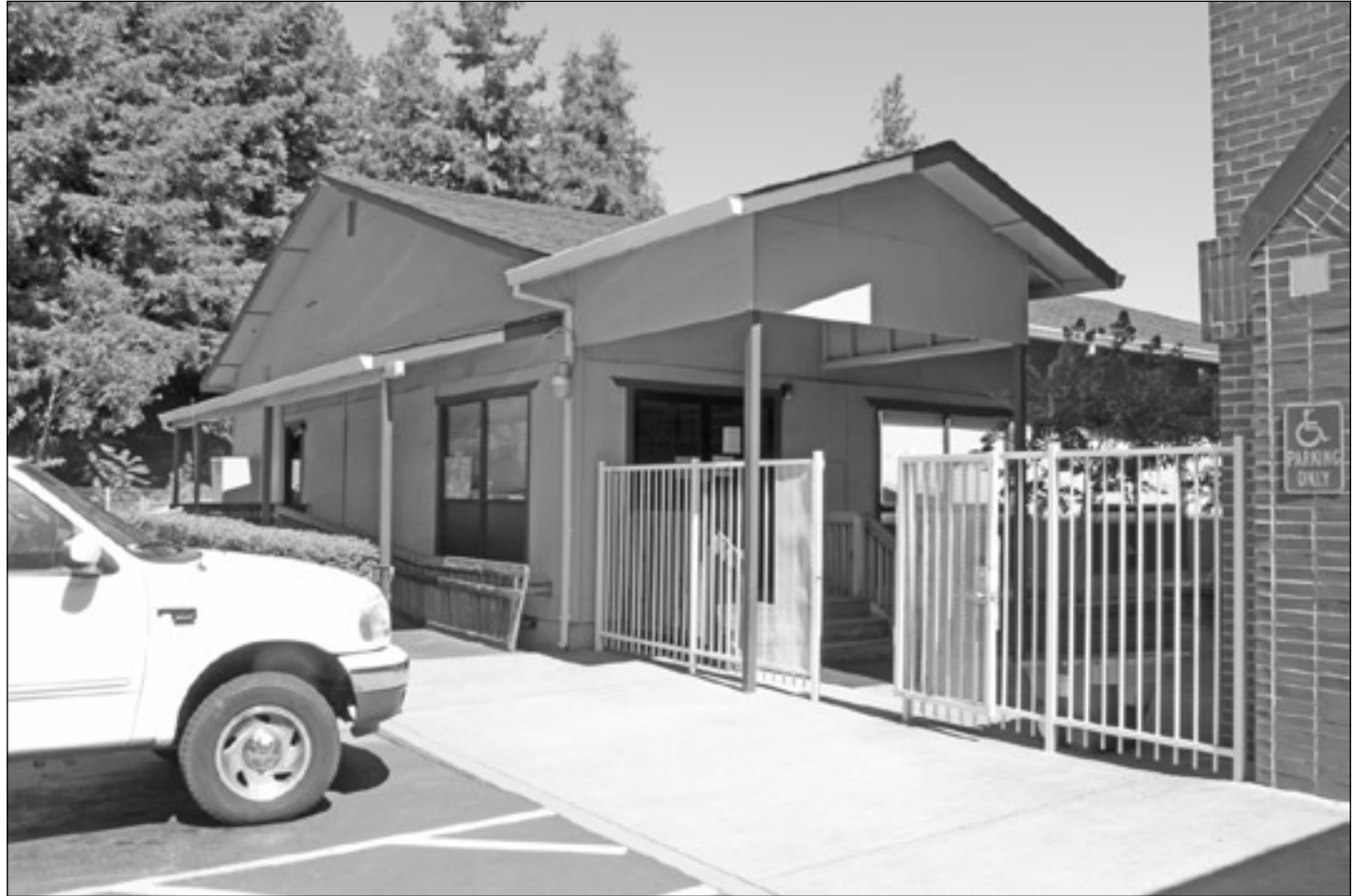
This building, which provided many preschool, childcare, after school and parent education programs during its 24 years of use, was replaced by the Alhambra Boulevard campus' new child development center. Photo courtesy, The Salvation Army
