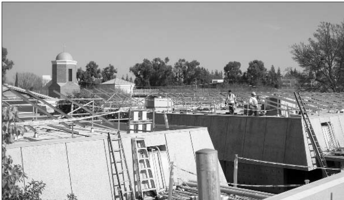
Photo courtesy, St. Francis High School SOLAR FARM TO SAVE ENERGY...AND MONEY. This photo shows the building of the solar "farm" that sits atop seven buildings at St. Francis High School in Sacramento. Photovoltaic panels were then installed on the frames. The completed system is expected to generate over one-third of the campus' energy, and is expected to save the school $1 million over the next two decades.
