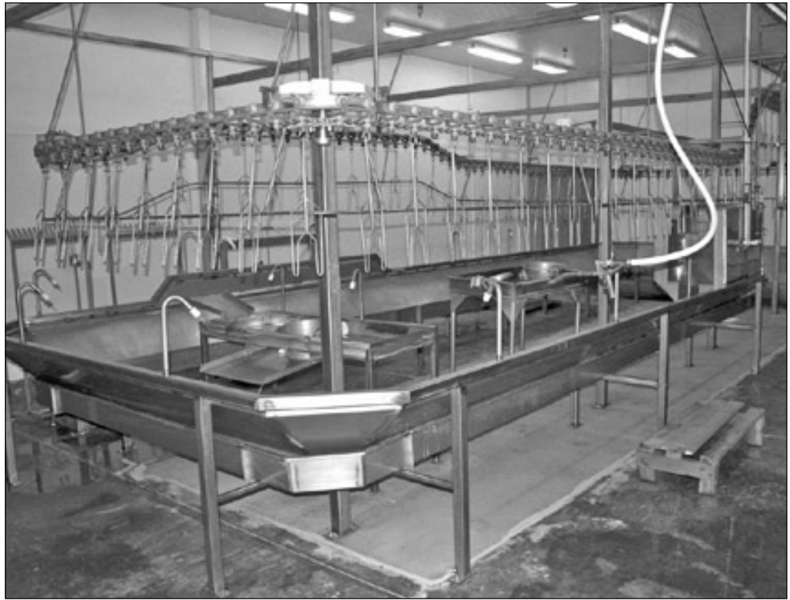
LARGER FACILITY. This large evisceration room is among the seven rooms at New American Poultry Co.'s new location.
