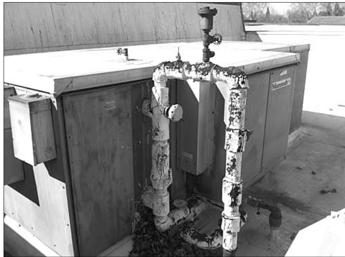
Photo courtesy of the Sacramento City Unified School District This is an inefficient 30 plus year old HVAC unit at California Middle School, which has gone well beyond its expected life cycle and should be replaced. With the passage of Measures Q and R, energy efficiency could go into effect.
