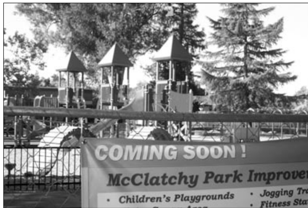
(above left) A fence surrounds McClatchy Park's under construction children's playground and tot lot. (above right) A worker places a stake in the ground near the new arch in front of the under construction McClatchy Park playground.
