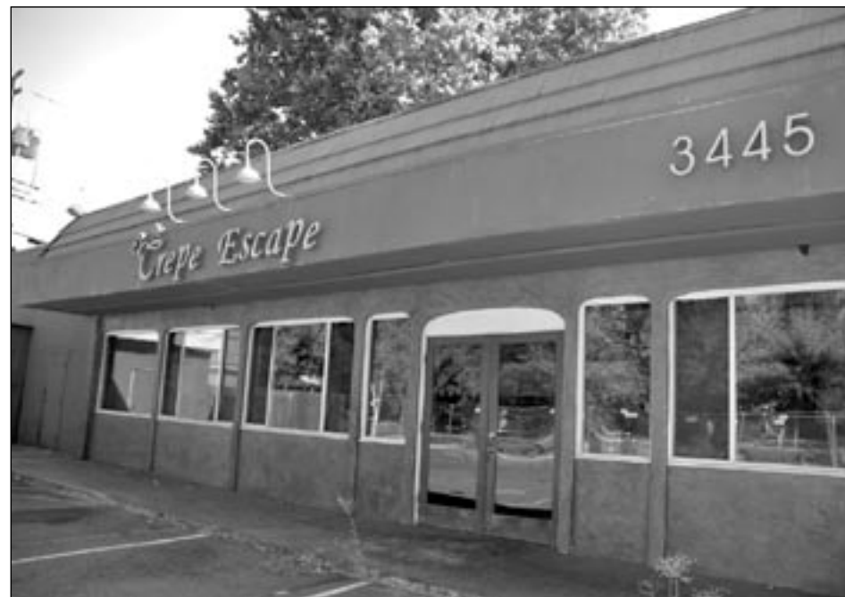
Boarded up Crepe Escape building.
