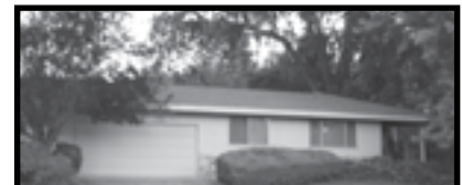
Duplex with Great Location Spacious duplex has 2 bed, 2 ba on each side. Private backyard patio & side courtyards, 2 car garage each side. Great investment property..... Call for more information Sindy Kirsch 730-7705
