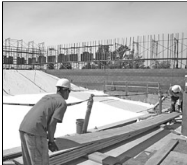
Pocket News Photo/Lance Armstrong Construction crew members work on the stage of the future performing arts center last week.
