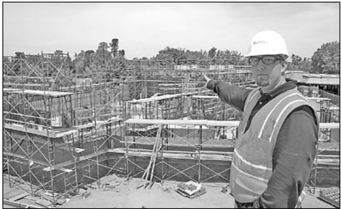
Pocket News Photo/Lance Armstrong Roebbelen Contracting Project Engineer Jeremy Wittmer stands above the under construction John F. Kennedy High School Performing Arts Center.
