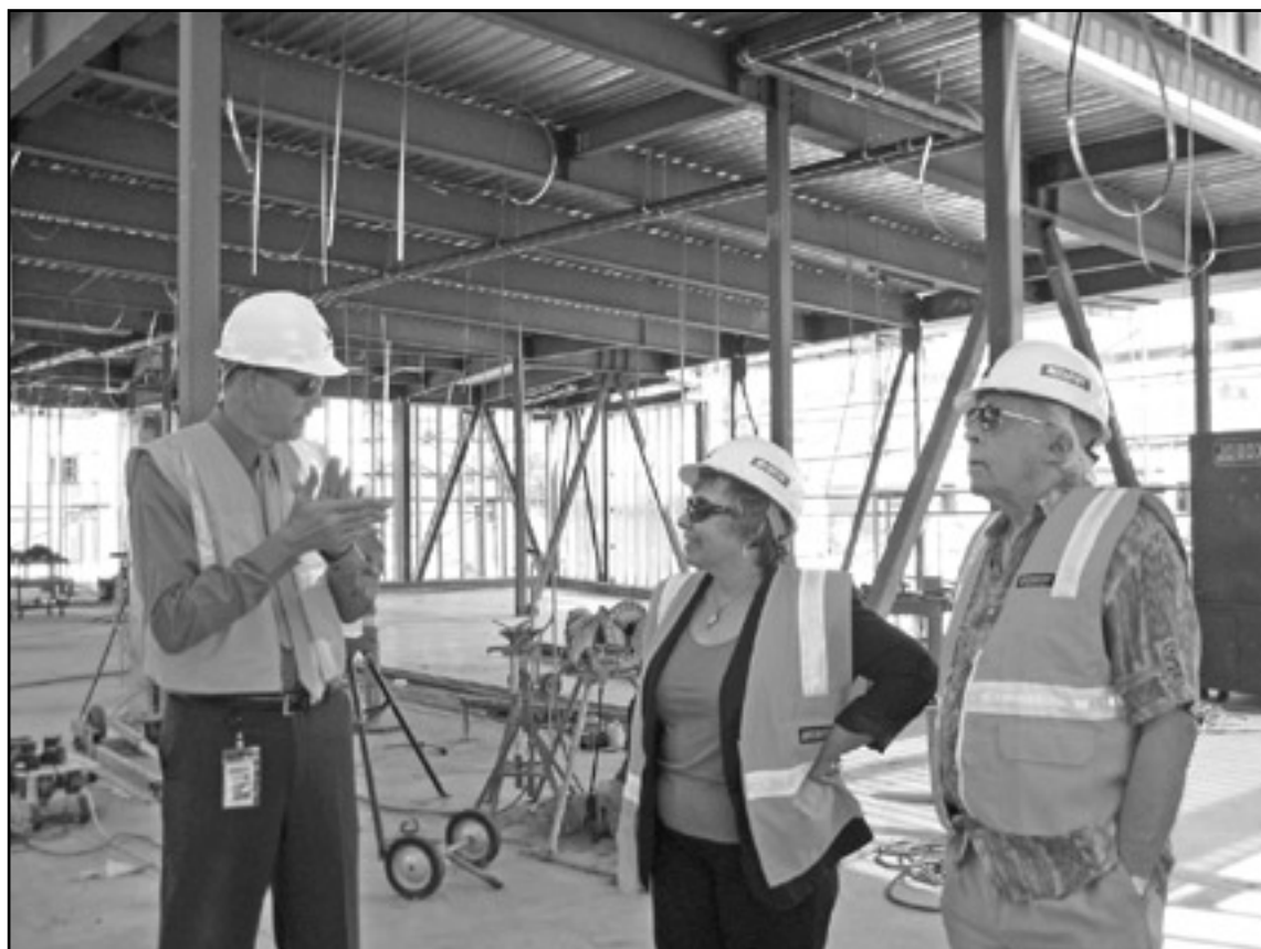
Photo courtesy Pictured here, Don Tucker, left, discusses the open space nature of the main area and the resulting high levels of natural daylight in the building with Director Sass and Councilmember Waters. The use of daylight is one of the energy efficiency features that qualifies the building to seek LEED Silver Certification. LEED stands for "Leadership in Energy and Environmental Design" and has three levels of certification for environmentally sustainable construction nationwide.
