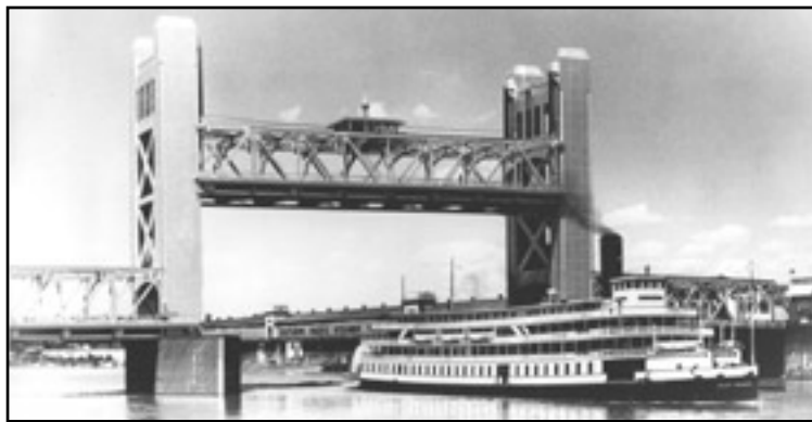
Photo courtesy of Sacramento Public Library, Sacramento Room The Delta Queen, the twin paddle wheeler of the Delta King, makes its way underneath the Tower Bridge in this c. 1936 photograph.
