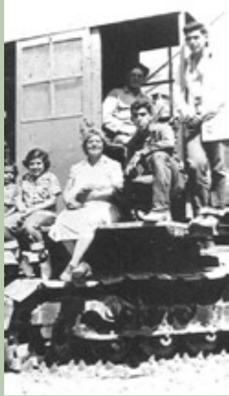
Building the Pocket, brick by brick
