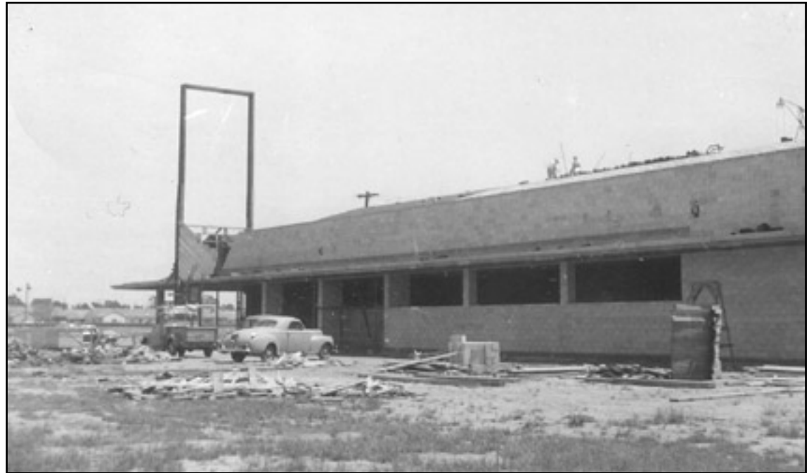
The Fernandez family was responsible for the construction of many residential and commercial buildings in the Sacramento area, including this Raley's supermarket at 2390 Fruitridge Road. The building is shown under construction in this 1953 photograph.
