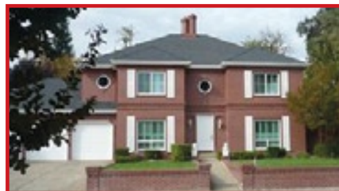
22 OAK RANCH COURT All brick home-not many of these in area. Home has been update extensively. Pictures don't do justice- must see! $1,100,000 SUSIE K. PARKER • 421-3546
