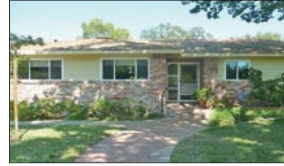
DEL RIO ROAD HOME
