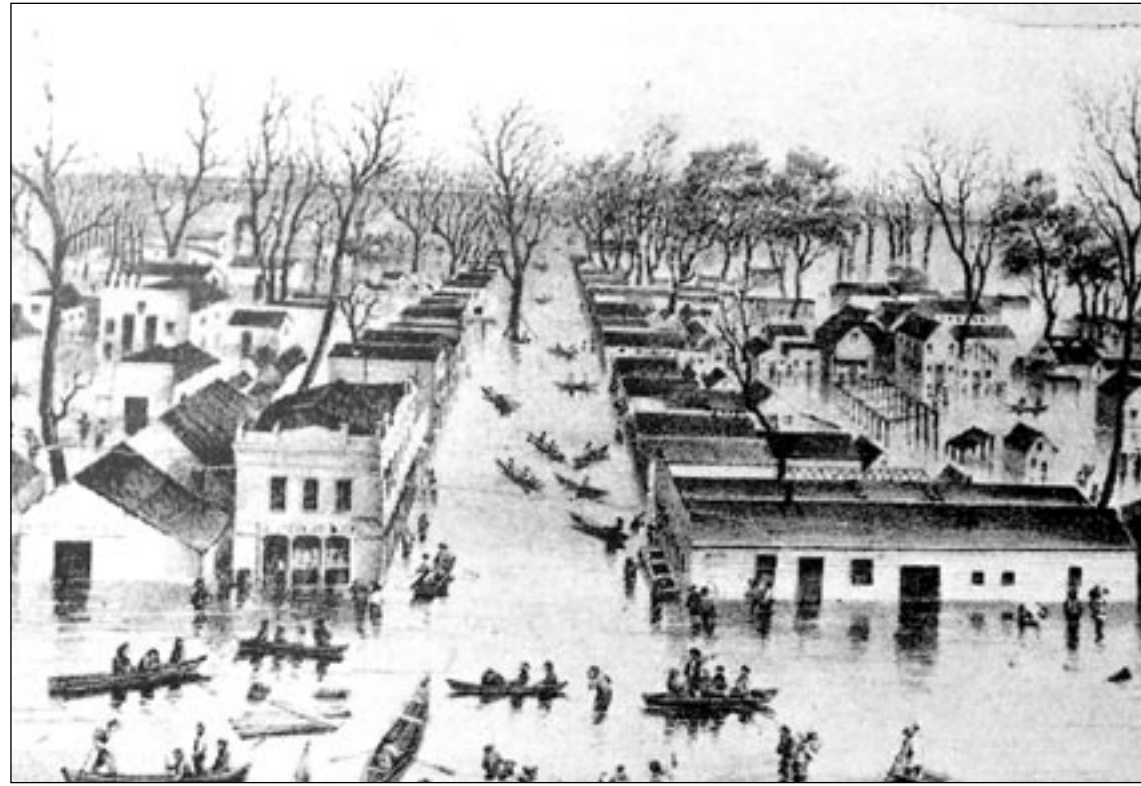
The flood of 1849-50 resulted in efforts that led to Sacramento City's notoriety as the "Levee City." Photo courtesy
