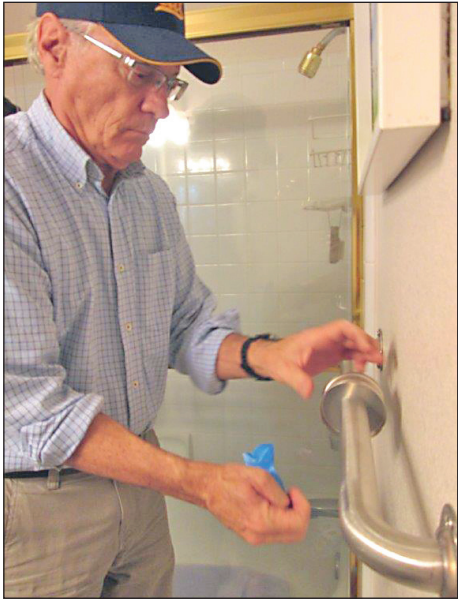
Photo courtesy Rebuilding Together Sacramento Rebuilding Together Sacramento volunteer installer Sandy Hanson works on putting in a grab bar at a local senior's home.
